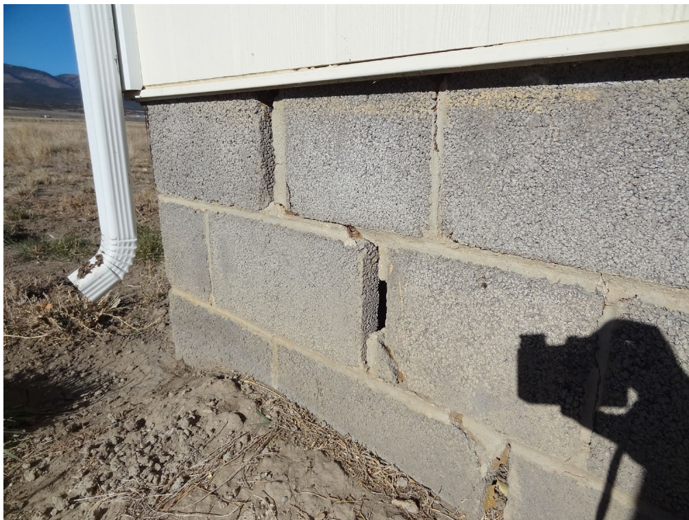
Steptoe Valley WMA Office - Building #2241 Description: CMU Foundation Repairs Needed.
